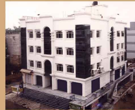
Aastha Trade Center , Bistupur Commercial complex Year: 2002-2003, Completed 30 crore
