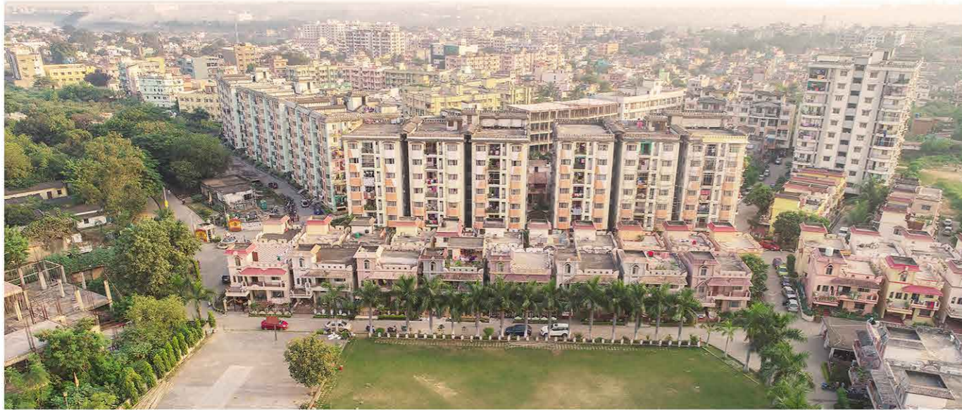
Aastha Space Town, Mango Residential complex & society Year:2004-2011, Completed & extention 80 crore
